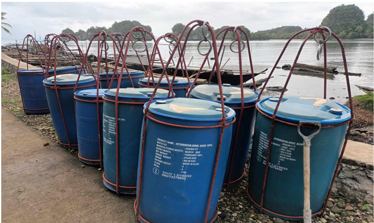
fabricated 16mm steel bar frame for 200L plastic drum
